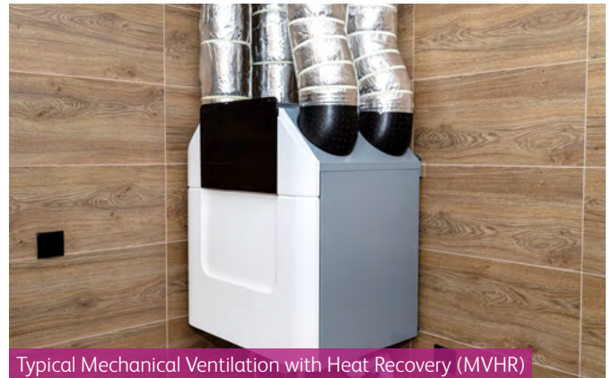
Typical Mechanical Ventilation with Heat Recovery (MVHR)
